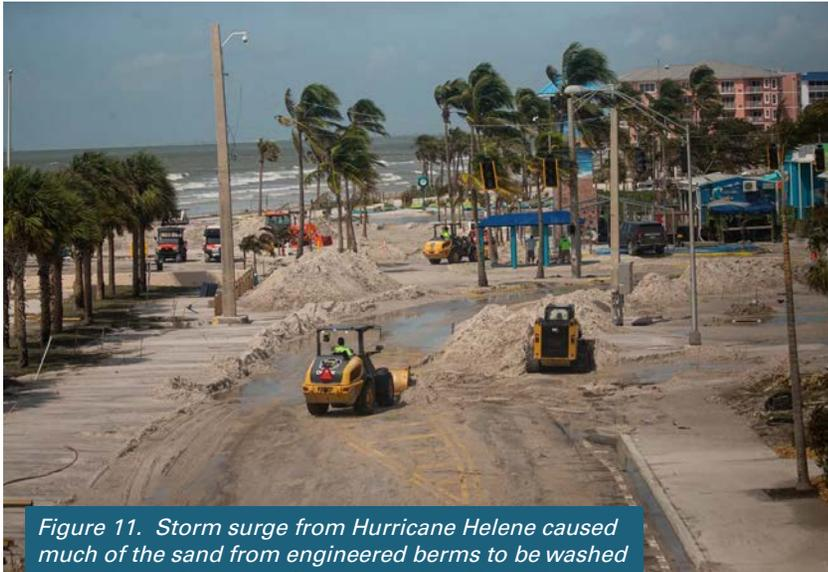
*Figure 11. Storm surge from Hurricane Helene caused much of the sand from engineered berms to be washed on to Estero Boulevard (source: Andrew West, The News-Press/USA Today Network, September 2024)*
