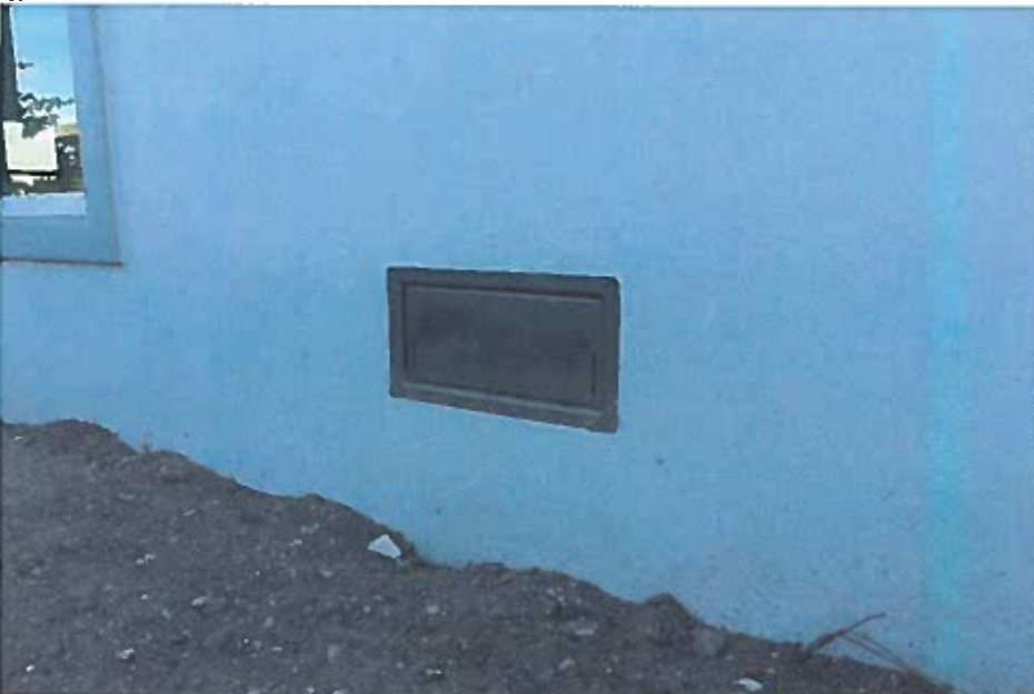
Typical Flood Vent 04/21/16
