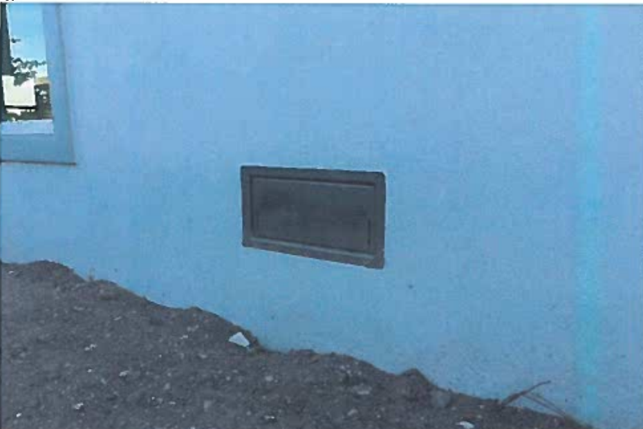
Typical Flood Vent 04/21/16
